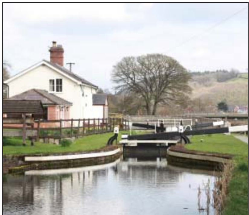
Waiting for the boats: Byles Lock, restored by SUCS
